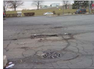
Asphalt Repairs
